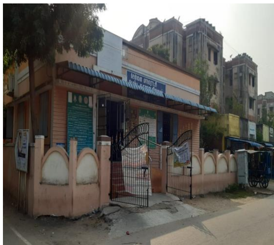
Image 14: PHC in AIR Site (Exterior)
